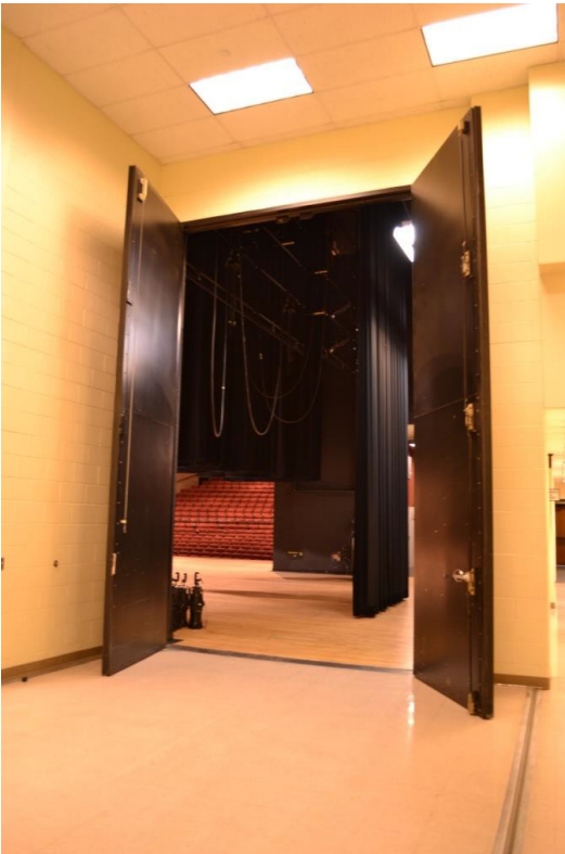
View of USR Loading Doors to Mainstage Theater Dimensions: 10' Wide by 16' High
